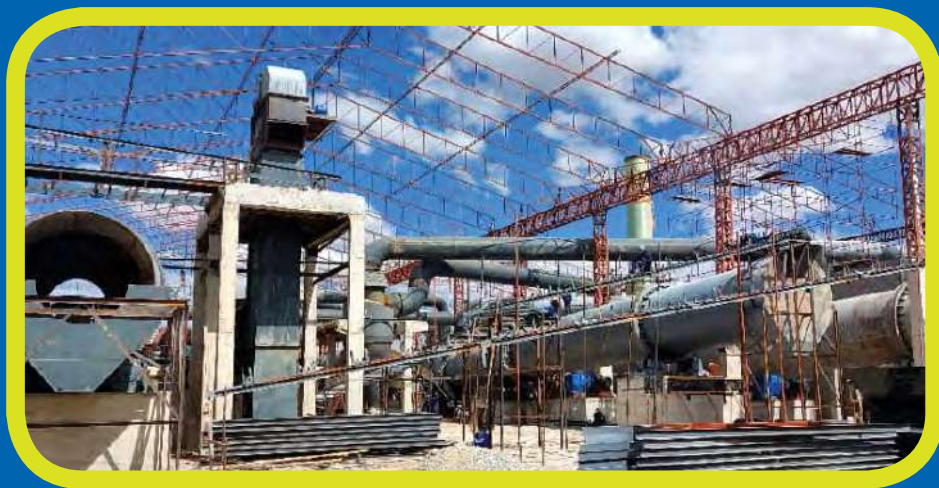
Ujenzi wa kiwanda cha mbolea cha ITRACOM Limited unaendelea eneo la Nala jijini Dodoma
